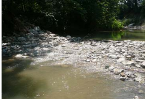
Rock riffles stabilizing the streambed.
