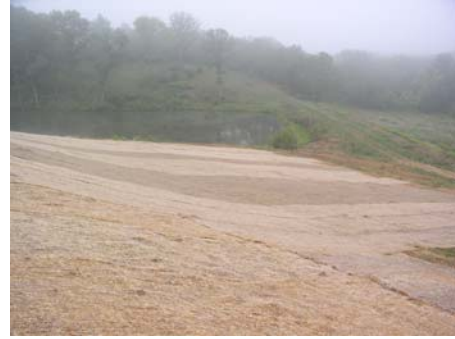
Erosion Blanket Installed
