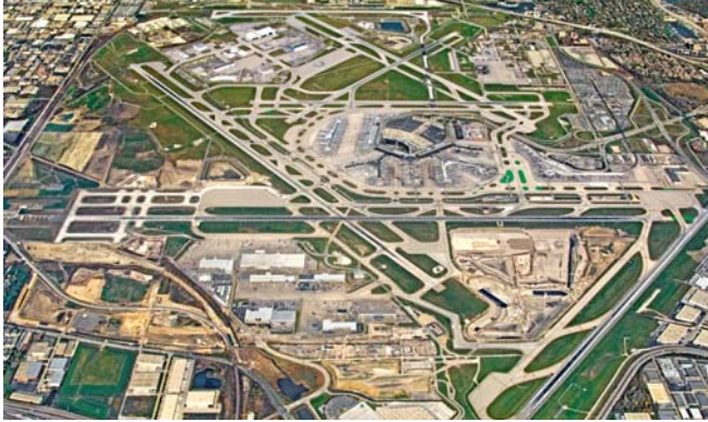
Aerial photo of O'Hare Modernization Program taken November 2008. Construction overseen by KDSWCD is located in the bottom left of the photo.
