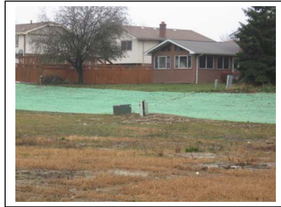
After: Completed treatment of disturbed area after application of excelsior blanket material
