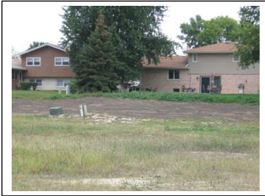
Before: Initial shaping of gullies extending upslope into adjoining residences
